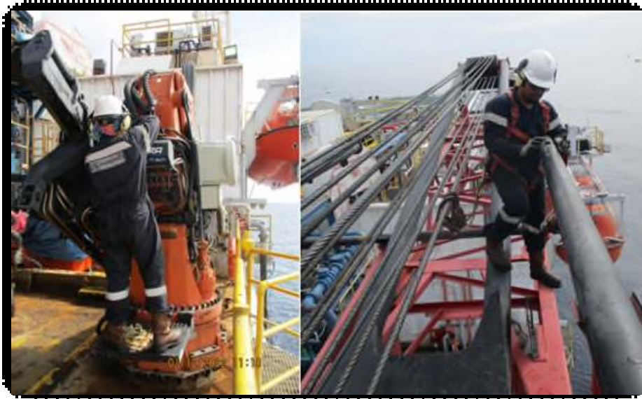
Vessel Deck Crane Inspection & Rectification
